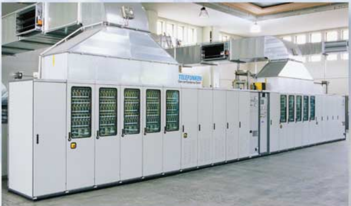
500 kW LW transmitter TRAM/P 500 L
